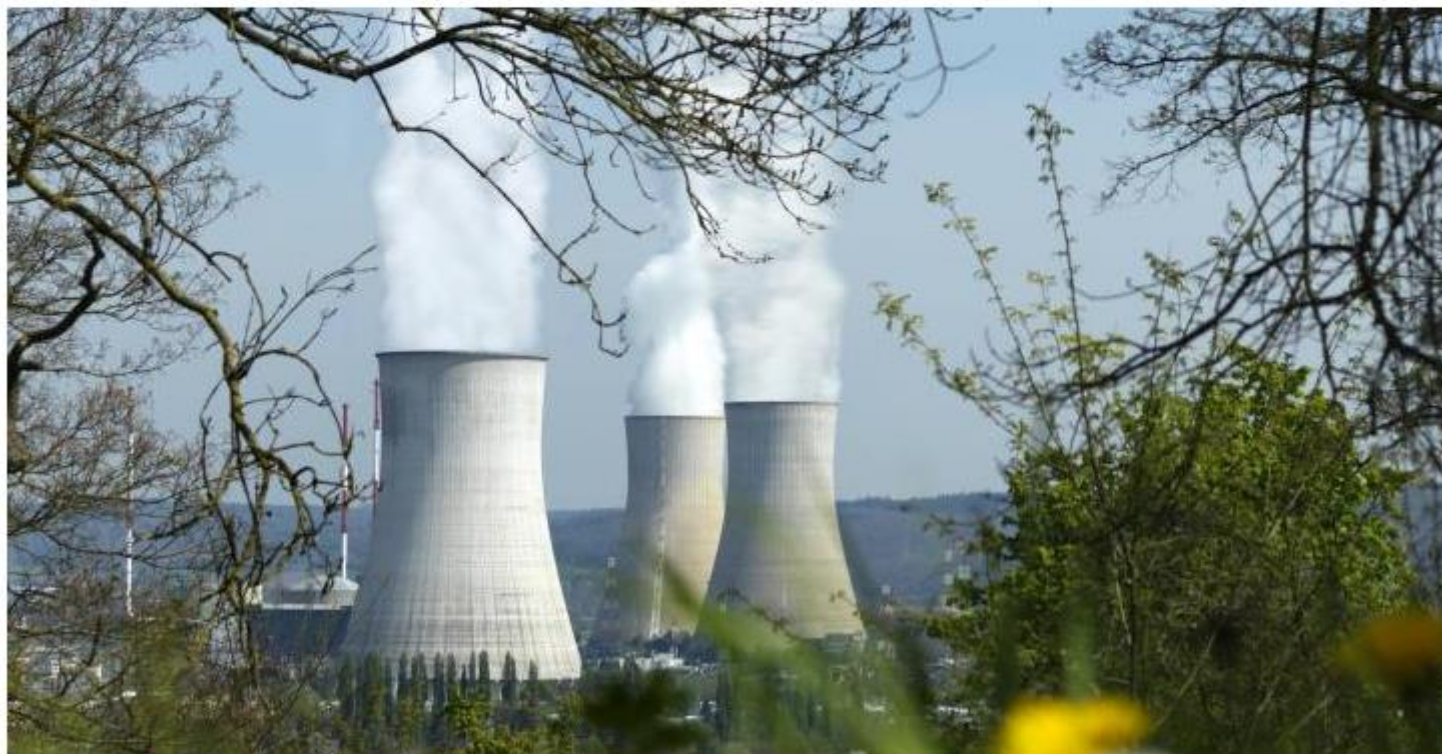
Belgian nuclear phase-out: Unit 2 of the Tihang power plant will go offline in 2023. (Image: Engie Electrabel)
